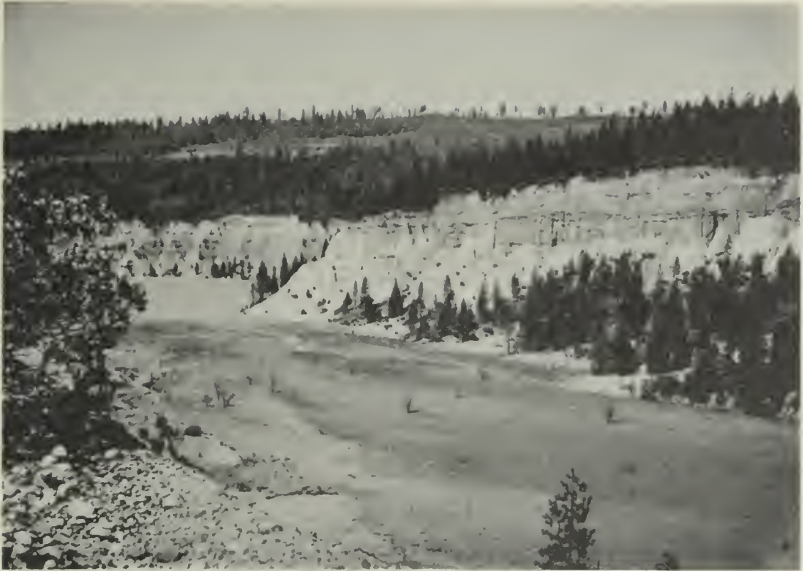
A, MALAKOFF HYDRAULIC PIT AT NORTH BLOOMFIELD, NEVADA COUNTY Gold was produced from gravel mined on a large scale from a Tertiary river channel until 1884, when an injunction obtained in Federal Court by agricultural interests practically put a stop to hydraulic mining. Photography, 1949; courtesy Thomas F. Ryder.
